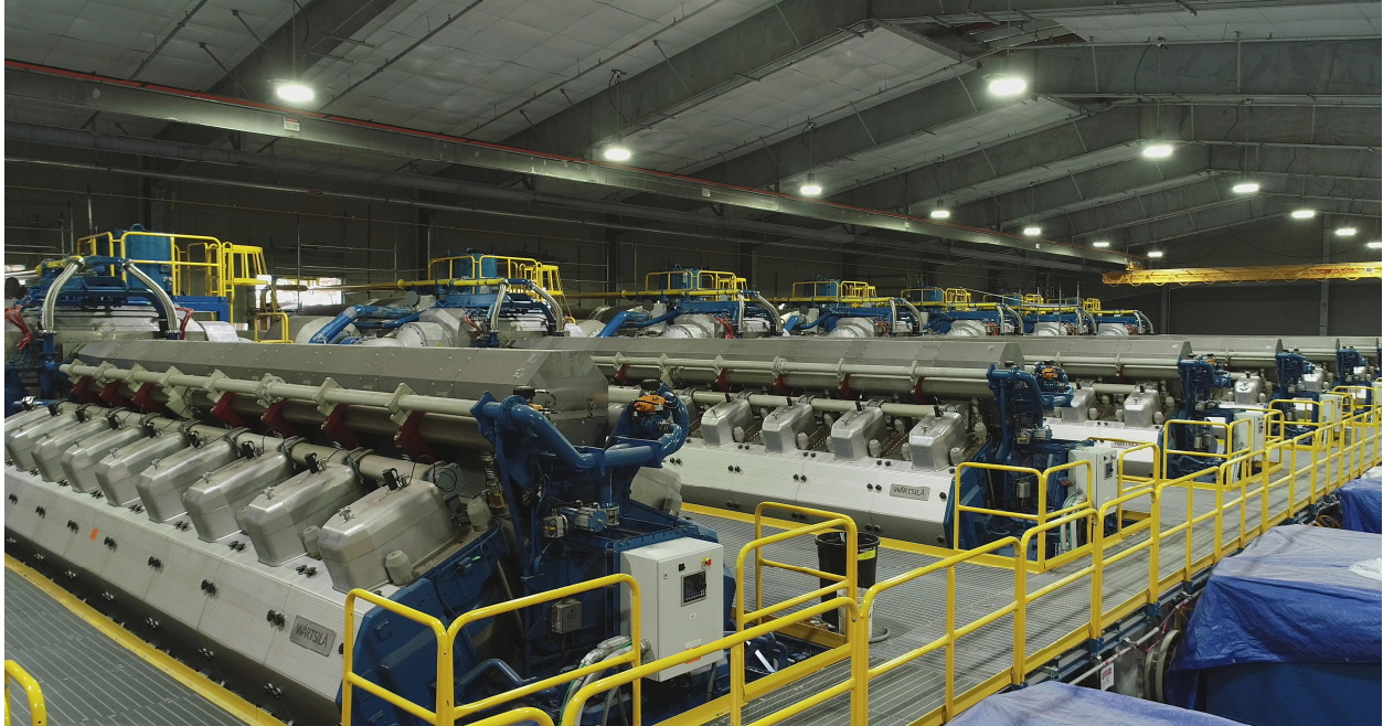
View Inside Engine Hall of NOPS Site (March 2020)
