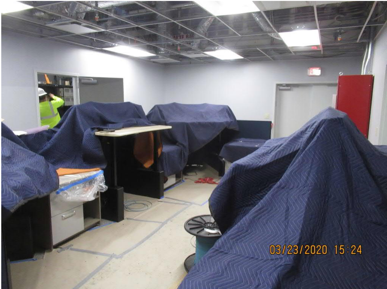
NOPS Control Room Furniture Install (March 2020)
