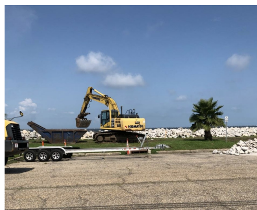
Breakwater Drive Completion date: Q4 2021
