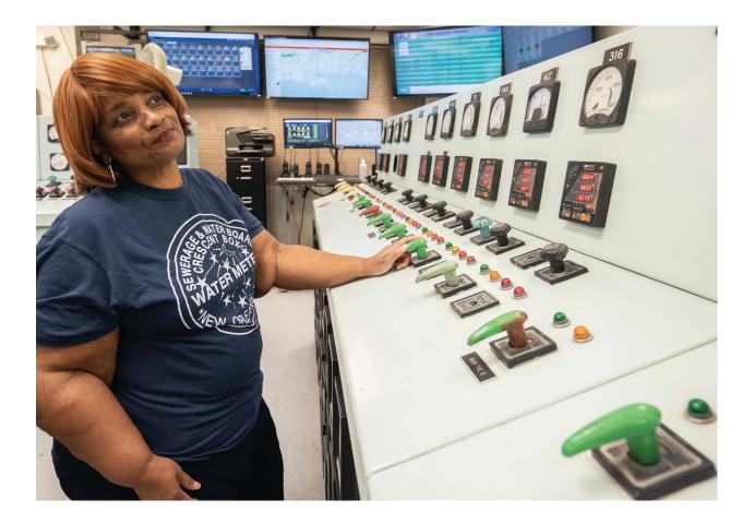
Our team works around the clock to make sure we continue to provide essential services. Here in Central Control, our employees are responsible for the delivery of an adequate supply of board- generated electrical power, the continuous monitoring of the operational status of all electrical switchgear and the testing of related electrical feeders and equipment.
