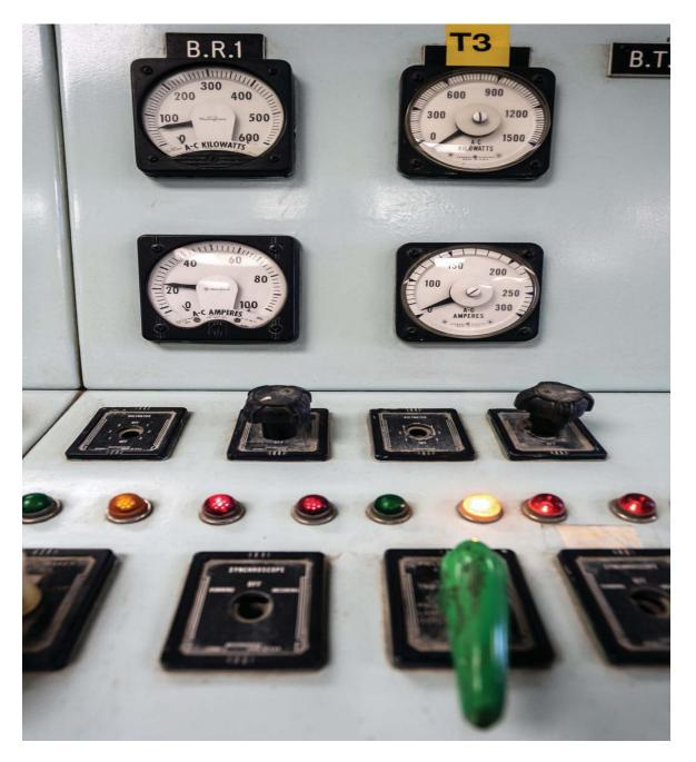
Of our 120 pumps, 51 run on an older frequency of electricity, 25 Hertz (Hz). We produce that power ourselves using steam turbine generators, frequency changers and Electro-Motive Diesel (EMD) generators. In all, we need about 52 megawatts (MW) of power to fully run the drainage system. We can produce more than 80 MW, giving us vital redundancy in our power supply.
